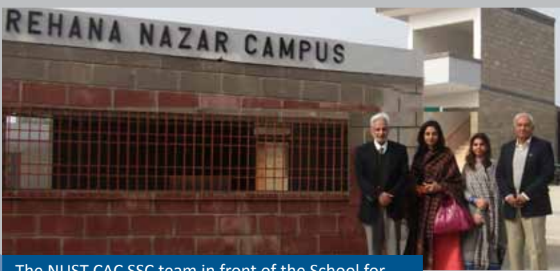
The NUST-CAC SSC team in front of the School for the deaf and dumb currently under completion
